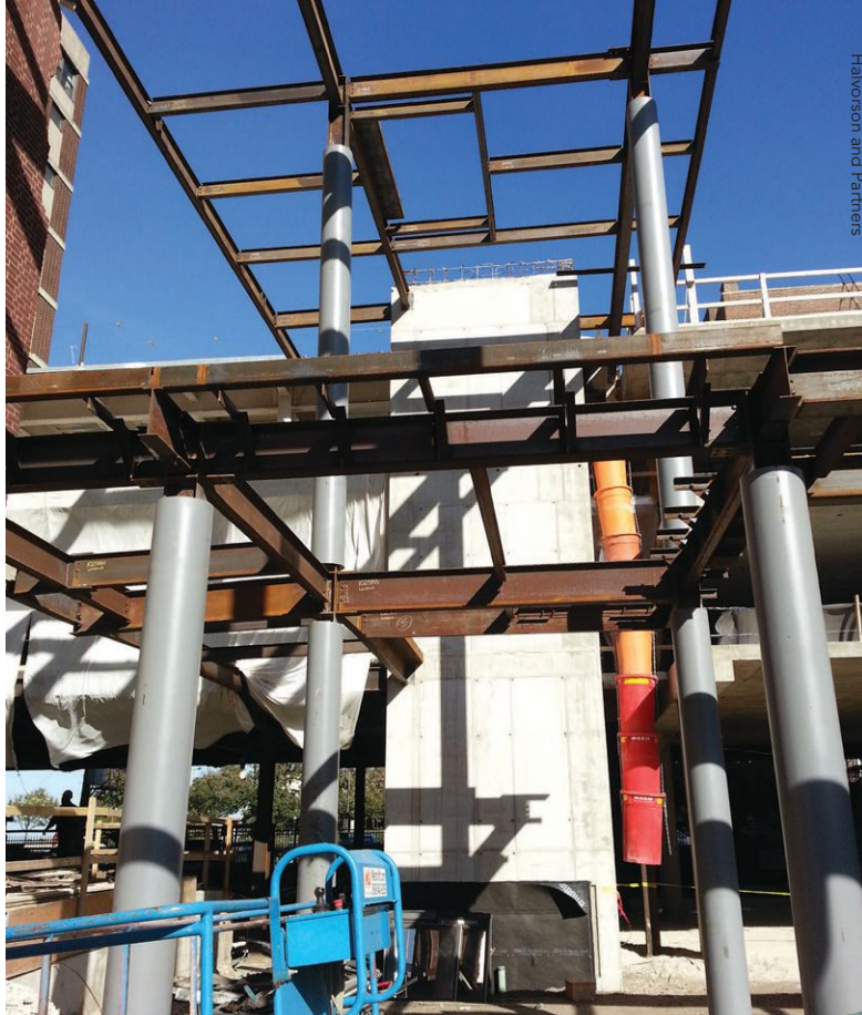
▼ Erecting the HSS framing for the Winter Garden.
